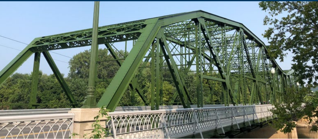
Broadway Bridge (Bridge 4930), City of St. Peter
