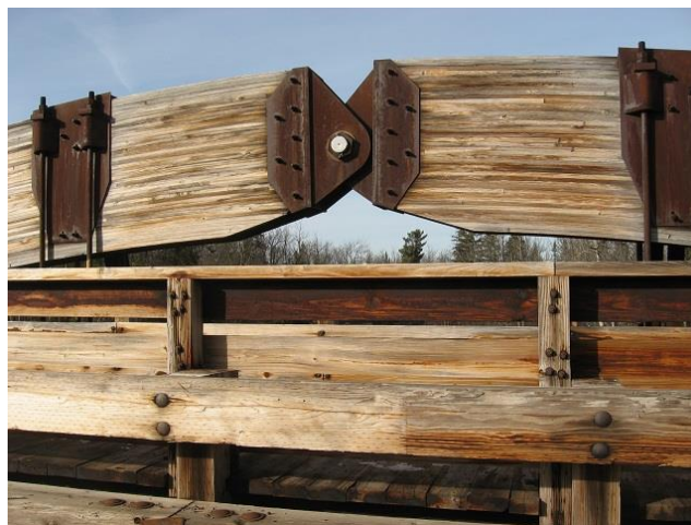
Graphic 3.1: Three-Pin Timber Arch Bridge, Hoyt Lakes, MN
