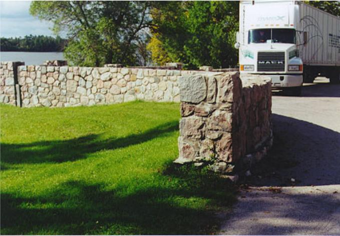
7. South curved Wall Section (note: vertical board at the far left pier is placed to partially cover the space between the corner joint)
