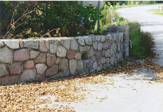
11. North Curved Wall Section (note: missing stone and overgrown vegetation along guard rail beyond)
