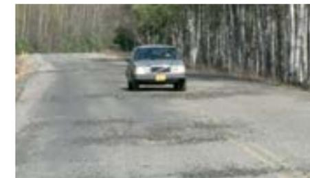
Frost action causes significant damage to roadways by expanding and thawing beneath pavement. It is the principal culprit behind spring potholes.
