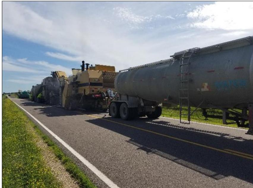
The CIR process involves a convoy of equipment to finish a road surface, including tankers that hold emulsion material and water, milling or crushing and recycling machines, pavers and rollers.
