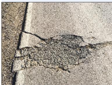
Freezing and thawing in pavement and the subsurface is a major cause of road damage.
