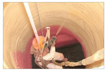
To prevent water from infiltrating manholes, sealants are sprayed on the inside and outside of manholes, and special gaskets are used between concrete sections.
