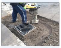
Effectively compressing the soil around a catch basin during construction prevents future settling and heaving.
