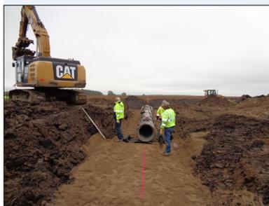
Road crews must prepare soil mixtures with care to ensure that seasonal weather and temperature change have little to no impact on movement at culverts and subpavement utilities.
