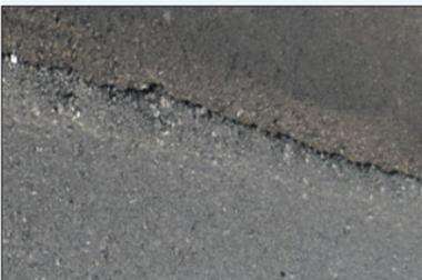
Low pavement air voids commonly occur where pavement sections meet, an area that is difficult to compact.
