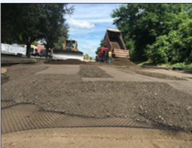
Added between pavement layers, geogrid increases the strength and durability of a finished road.
