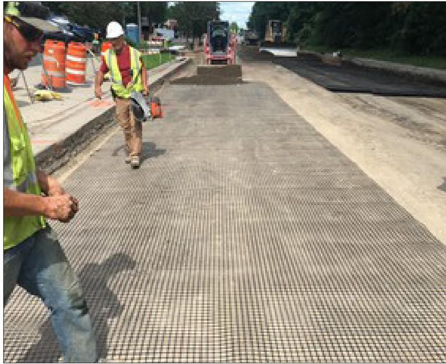
The synthetic geogrid material comes in rolls, allowing the material to be easily placed over an aggregate subgrade.
