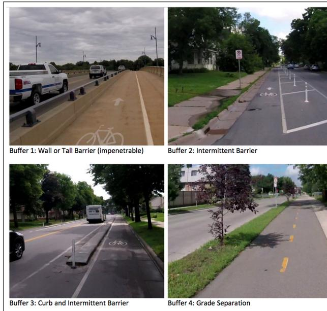
Four separated or buffered bike lane designs, shown at left, were included in the online user survey about bike lane preferences. The lanes’ separation strategies ranged from intermittent flexible posts (top right) to a complete grade separation from the main roadway (bottom right).
