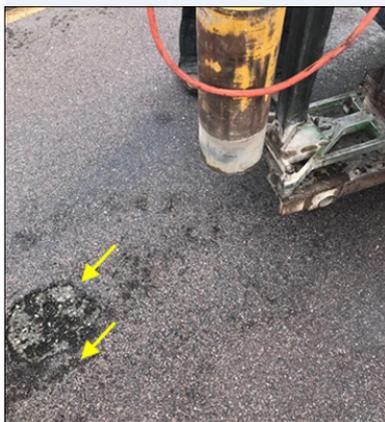
Researchers identified partial stripping of the seal coat on this asphalt pavement.
