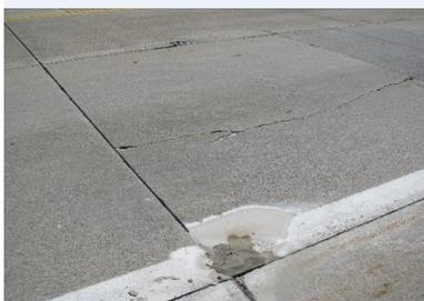
This overlay at a site in Michigan shows corner damage and midslab longitudinal cracking.
