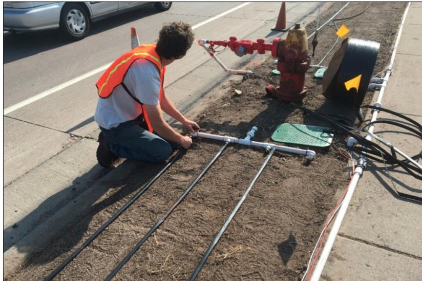
Drip irrigation systems were installed on turfgrass test plots on several boulevards with fire hydrants as the water source. The systems included connectors, valve controllers and timers attached to the hydrant.
