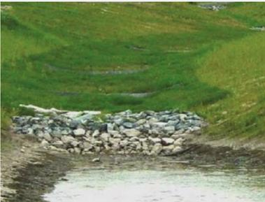
Two bioslopes lead to a bioswale. Stormwater follows the bioswale and is filtered through a stone outlet into a detention pond.
