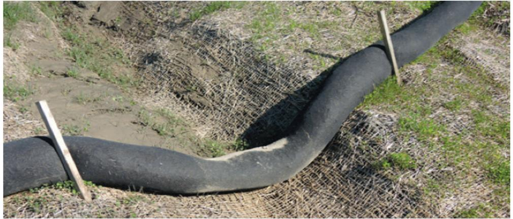
Overtopping occurred at this failed SCL installation, indicated by the dried sediment on the log.
