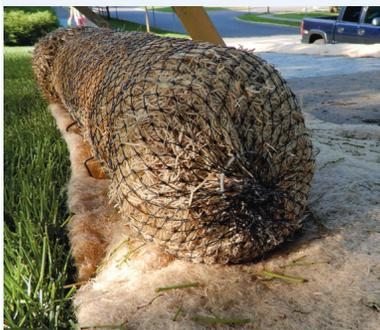
This SCL was correctly installed on a wood fiber blanket. A wooden stake on the downslope side of the log prevents it from rolling.
