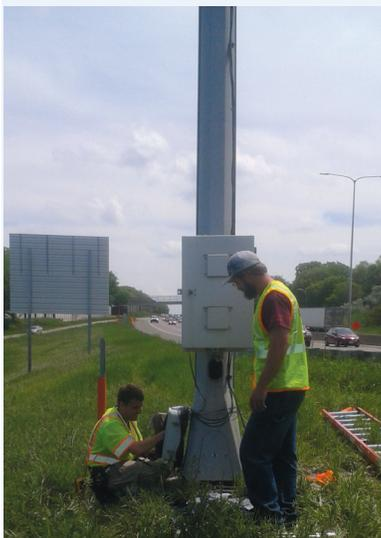
Speed detection sensors were installed on poles every half-mile through a new highway construction work zone.
