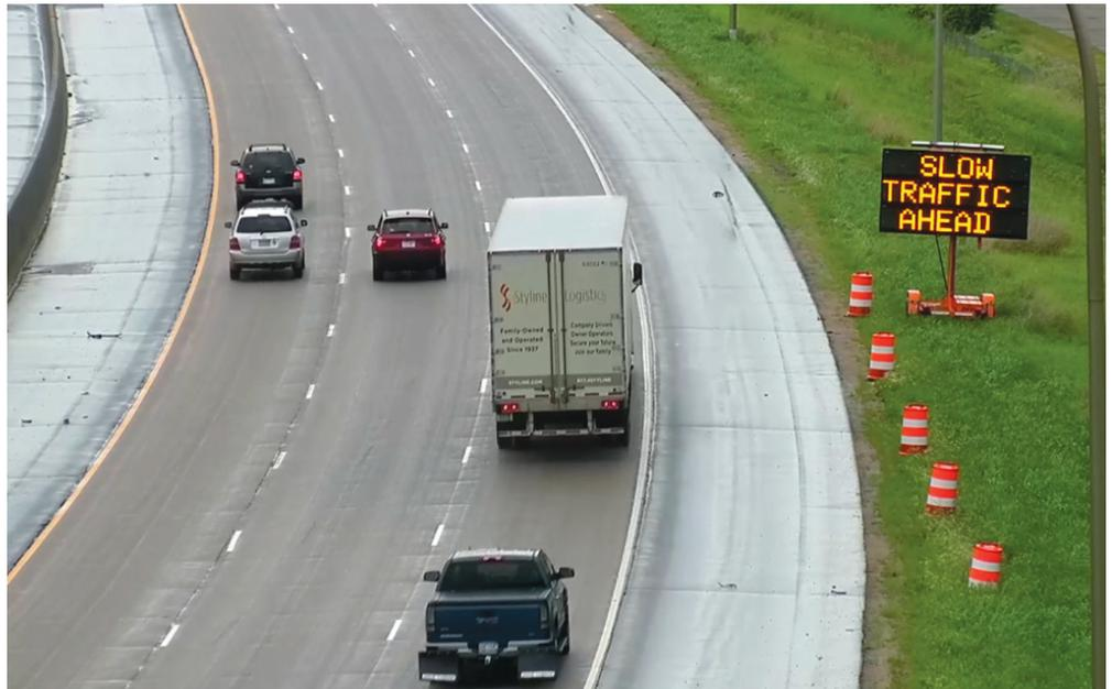
A variable message sign, part of the SWZSN, displays the warning “Slow Traffic Ahead” in a construction zone.
