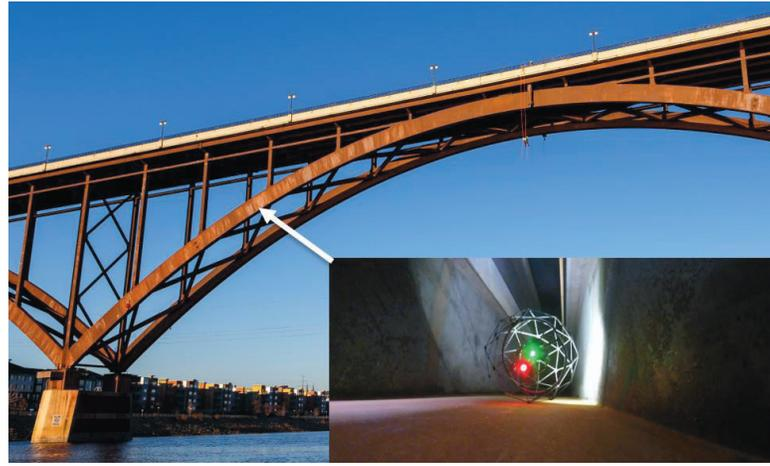
Bridge inspectors used multiple UAS, including a new drone that flies within a cage that can roll in confined spaces, preventing collision damage.
