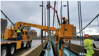
Using a "snooper" truck during a bridge inspection requires closing at least some lanes of traffic.
