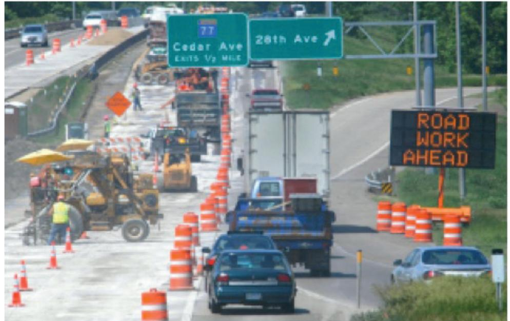
A challenge in designing a work zone layout is to clearly guide motorists around or through the zone with sufficient approach to allow drivers to reduce speed and understand where to go.
