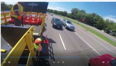
In a common type of close call, the dark car shown here fails to merge until it is too close to the work zone, forcing the silver car out of its lane.
