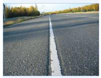
After only two years of service, this pavement marking has significantly deteriorated, demonstrating the importance of using products with longer service lives.
