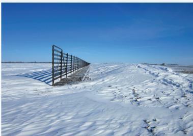
Man-made materials can be used to build effective fences for capturing blowing and drifting snow alongside agricultural fields, keeping roadways clearer.
