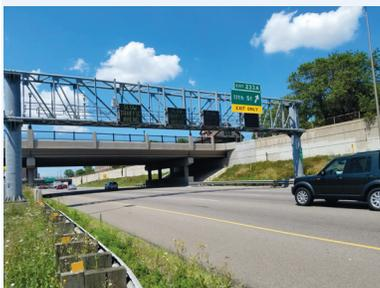
To deploy the ATM system, MnDOT attached two sets of changeable message boards to gantries above the freeways.
