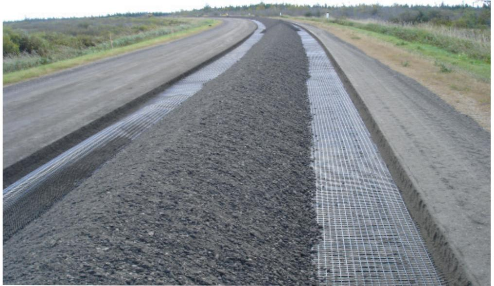
Sandwiched between aggregate base layers, geogrid matting stabilizes and stiffens aggregate base courses, strengthening pavement over soft subgrades.
