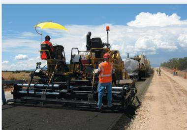
CIR involves pulverizing a surface layer of pavement and mixing it with an emulsion to create a new layer of asphalt.
