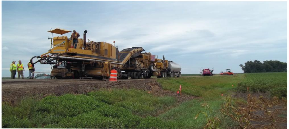
CIR trains like this one allow crews to grind up the top few inches of a pavement, mix the material with new bituminous material, and lay the new mix down in one pass to provide a long-lasting, new asphalt structure.
