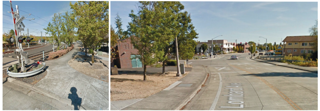
The light rail station in Beaverton, Oregon, a Portland suburb, has very high light rail ridership but doesn’t have a terminal or park and ride, and doesn’t stand in a central business district.
