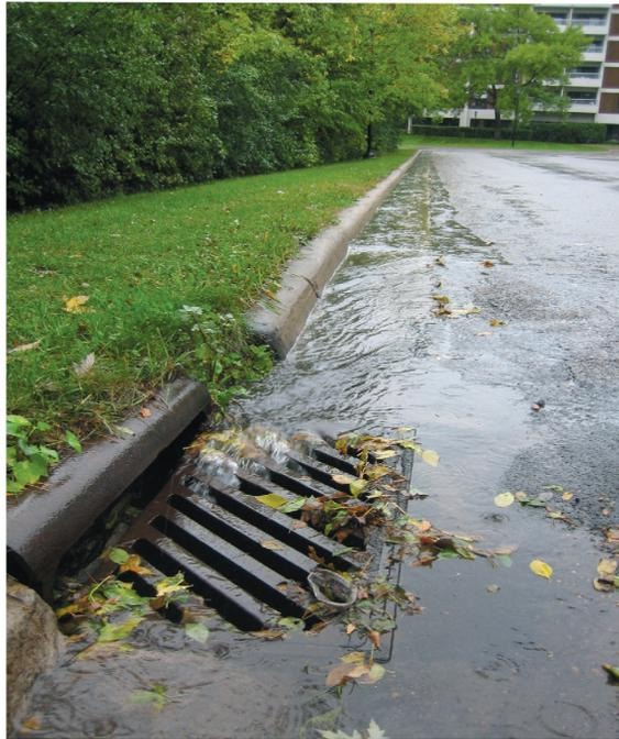
Unlike a sidewalk, the street is part of the watershed’s EIA, which represents a portion of the TIA and is a better parameter for establishing stormwater control measures than the TIA.
