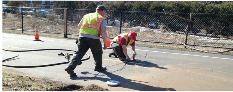
Inductive loops, which consist of three to five turns of loop wire embedded in a channel cut into pavement, are suitable for permanent counts, but they must be calibrated to detect bicycles.
