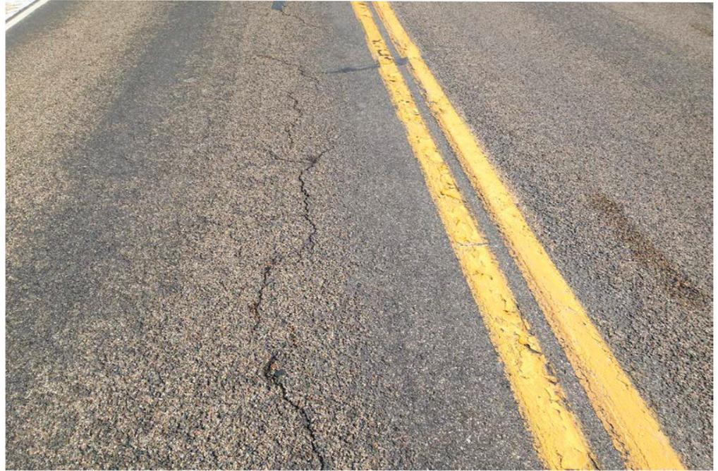
After 15 years of study, researchers began to see marked differences in deterioration between test sections, including wheelpath cracking in subsections of section 1.
