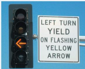
Flashing yellow arrows can increase intersection safety and efficiency.
