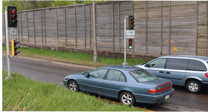
The improved ramp metering algorithm responds better to live road conditions by reacting to vehicle density rather than traffic flows, which reduces the number of meters operating on light traffic days.
