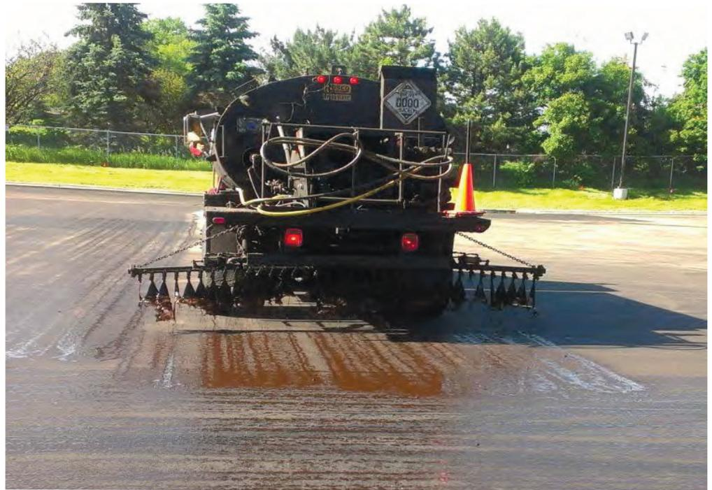
Applying a tack coat during paving helps to bind layers of asphalt together. Inadequate binding can lead to premature pavement distress, potentially reducing service life of some Minnesota pavements by up to 25 percent.
