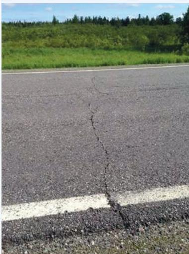
Poorly performing asphalt pavements motivated laboratory tests to predict the behavior of MnDOT's asphalt mix designs.
