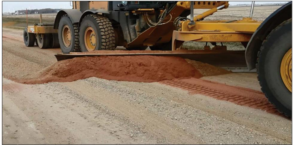
Researchers used motor graders to blend crusher dust with loose aggregate floating on the road surface. This was intended to restore fines that bind the aggregate. The effectiveness of the procedure depended on the plasticity of the available crusher dust.
