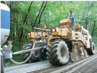
Mixing cement into subgrade soils increases their stiffness, strength and durability.
