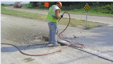
After removing damaged concrete, workers air blast excess material before applying a partial-depth repair patch.
