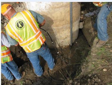
On the Minnesota River Bridge, MnDOT personnel installed tethered switches buried in the soil near piers.
