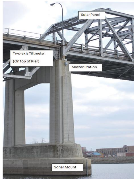
On the Winona Bridge, sonar and tiltmeter data are relayed to a master station for wireless transmission. The system is powered by a solar panel.
