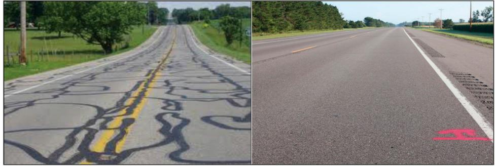
Pavement preservation activities should be undertaken before significant distress is visible. Distress in the pavement on the left is too significant for preservation to be beneficial, while the pavement on the right is a good candidate for preservation.
