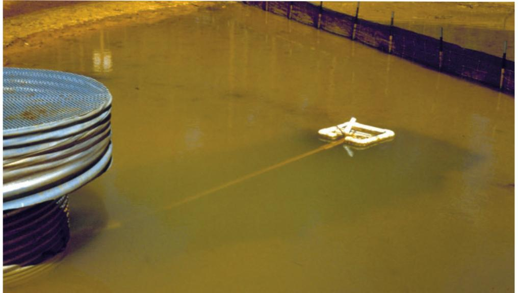
Floating-head skimmers in temporary stormwater ponds, including the Faircloth skimmer shown, use gravity to drain the cleanest water from just below the surface of the pond while sediment settles to the bottom.
