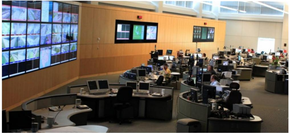
From the RTMC’s control room, engineers can monitor and manage Twin Cities freeway traffic using data from thousands of in-pavement sensors.
