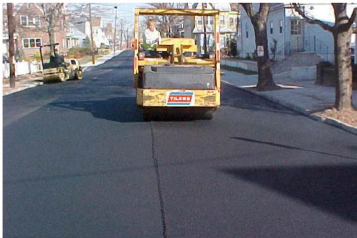
The final report for this project includes detailed advice about the construction of composite pavements, including roller placement for proper compaction of asphalt overlays at longitudinal joints.
