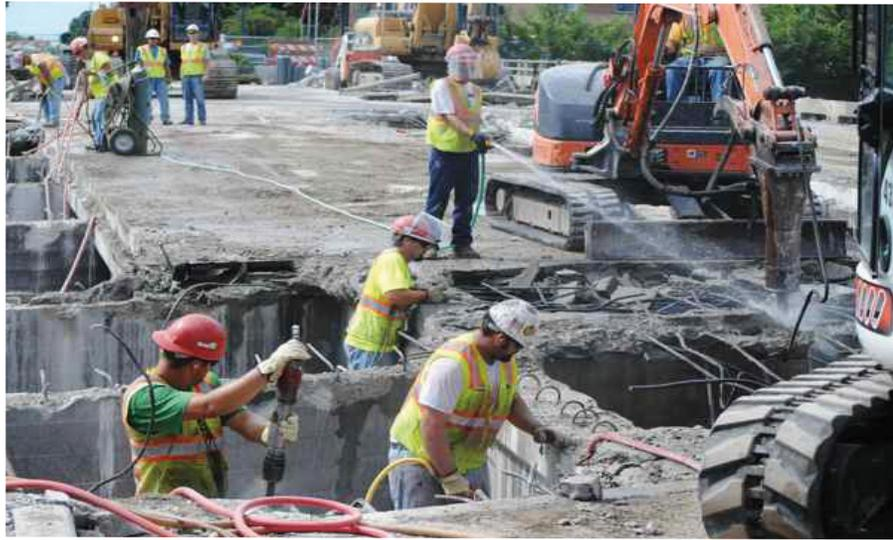
Water spray keeps dust down during concrete bridge deck removal, but has the potential to create high volumes of slurry that must be controlled to protect waterways.
