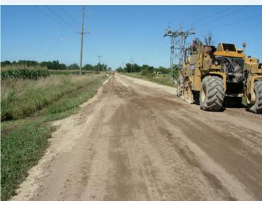
Self-cementing materials such as fly ash are mixed into subgrade soils to strengthen and stiffen them.
