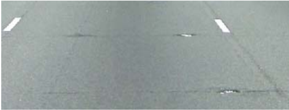
Figure 7: I-394 (EB) section, photo taken summer of 2008.
