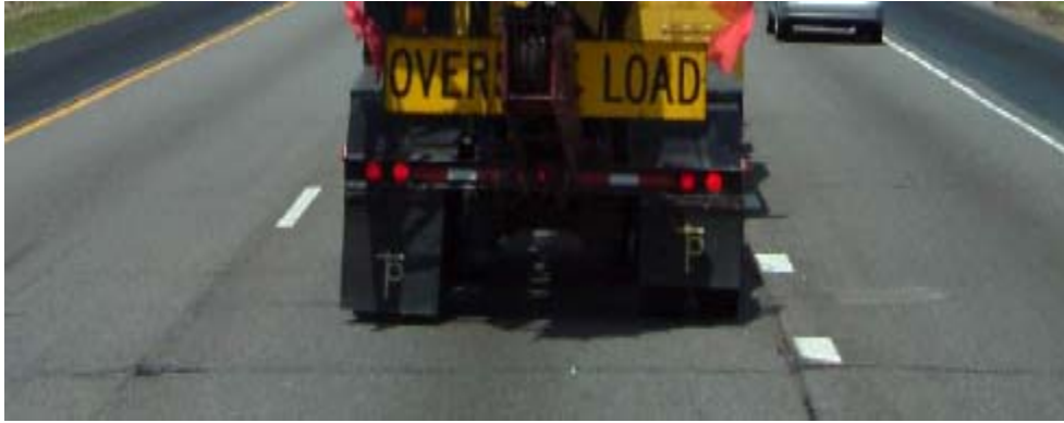
Figure 1: Transverse joint deterioration, photo taken summer of 2008.
