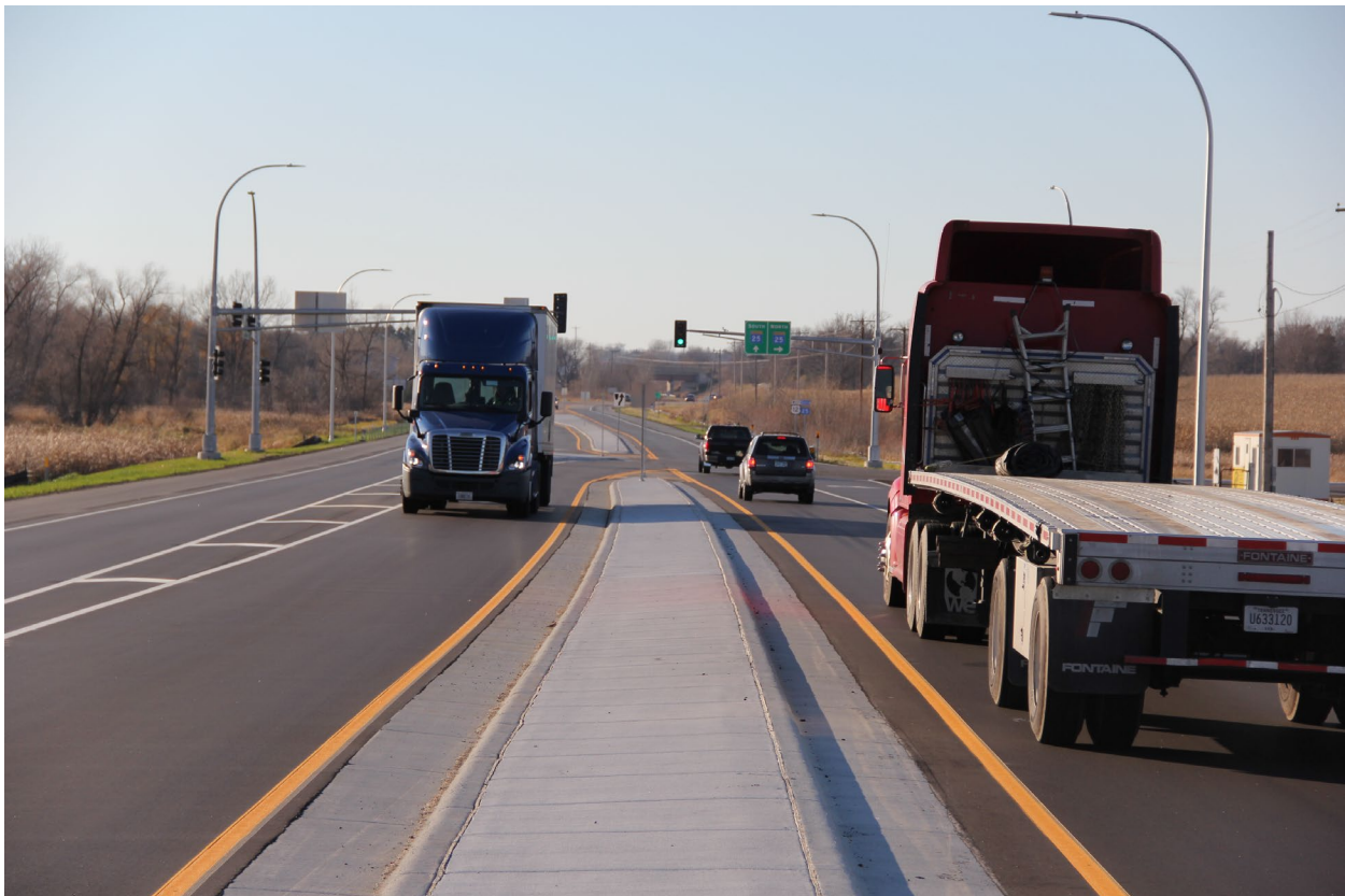
Trucks traveling on MN Highway 25. Source: MnDOT District 3 Staff
