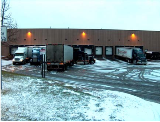
Figure 2-2. Terminal with inadequate maneuvering and parking space
