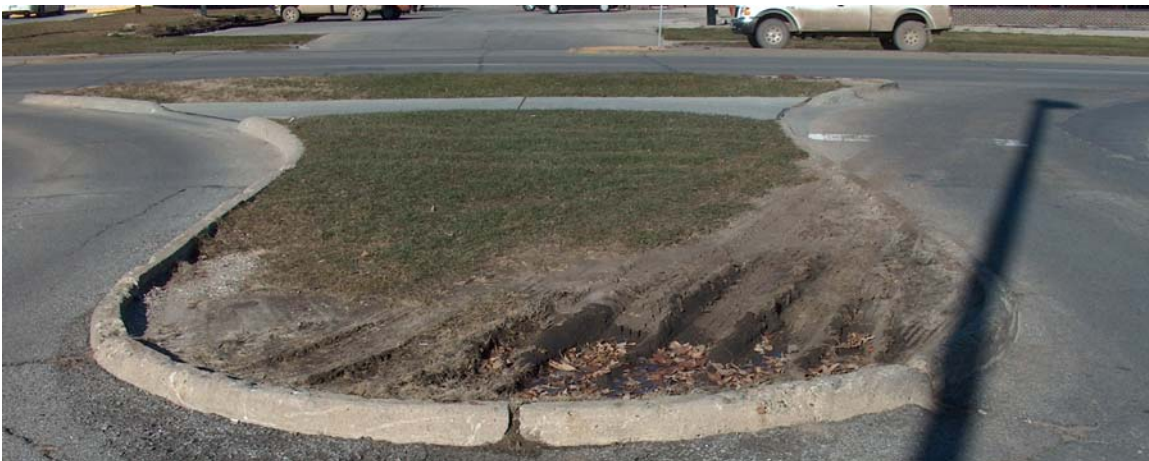
Figure 2-1. Wheel ruts in a median with an inadequate turning radius for trucks
