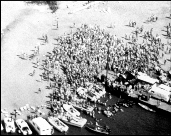
Figure 3.14 Dredging Material Beach
