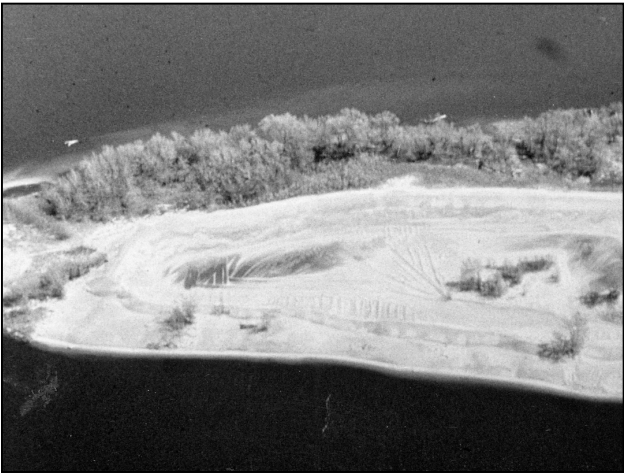
Figure 3.13 Dredging Material Island
