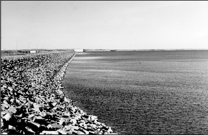
Figure 3.9 Typical levee structure
