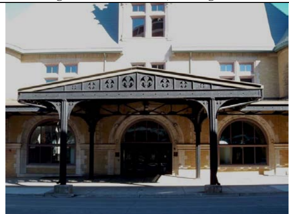
Michigan Street main entrance, looking east
