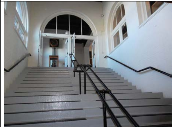
Main stairwell to track level, looking up toward great hall
