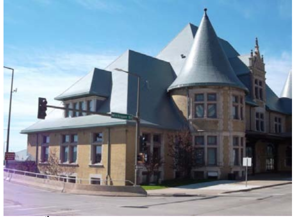
5 th Avenue elevation, looking southeast
