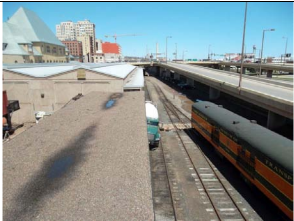
From parking deck, looking north
