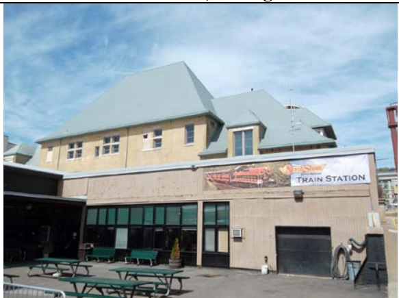
Amtrak wing at track level, looking west
