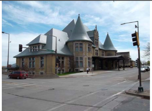
Michigan Street elevation, looking southeast
