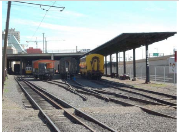
Canopy and parking deck, looking north
