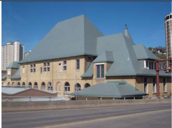
5 th Avenue elevation, looking southwest
