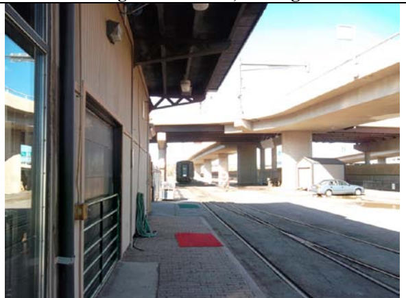
Railroad tracks east of train shed, looking north
