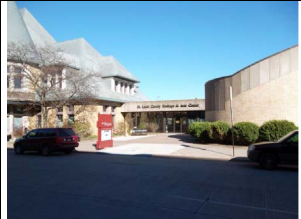
Connection with performing arts wing, looking east
