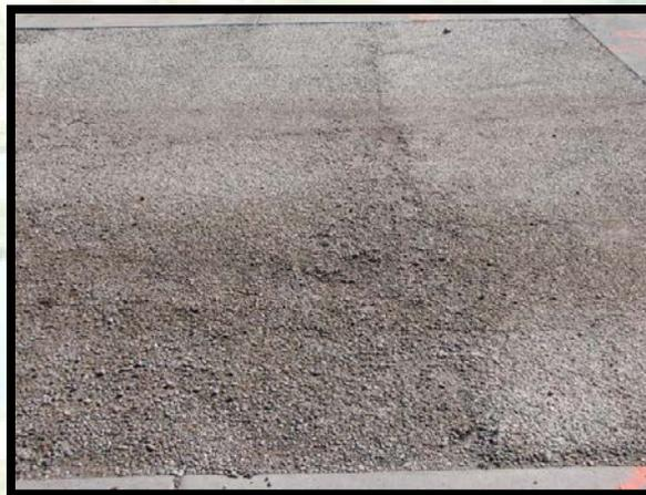
A large longitudinal crack also propagated down the length of the driveway, and was likely a result of FWD testing, traffic, and thermal loading.
