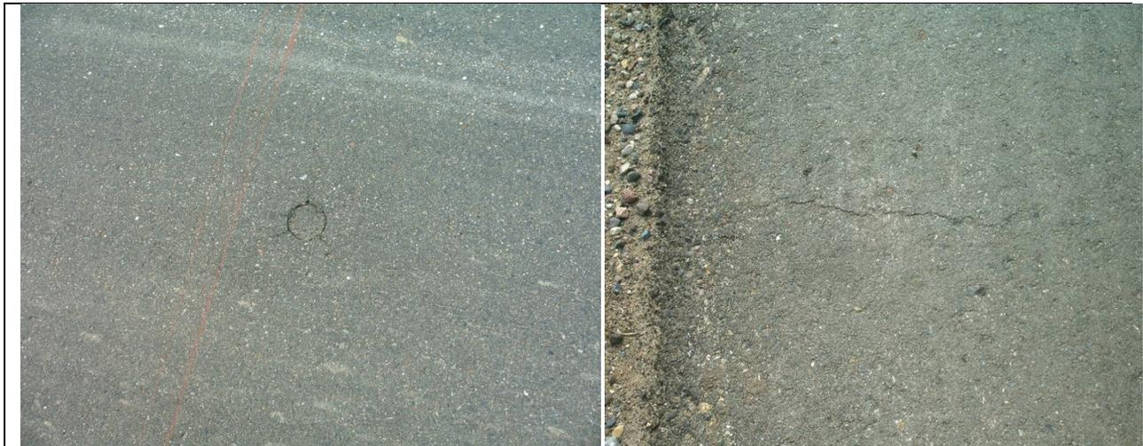
Figure 5.3. Hassan Township: Coring (Left) and Transverse Cracking (Right), March 2008
