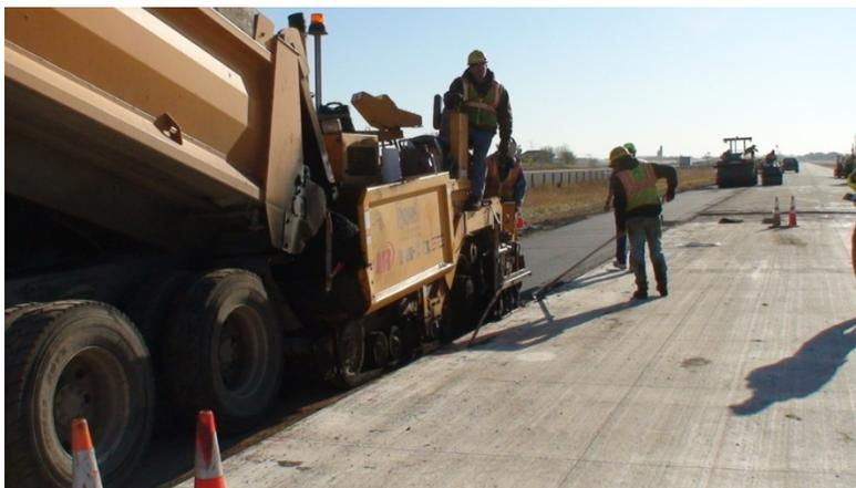
Figure 5.6. MnROAD MWSS Shoulder Construction
